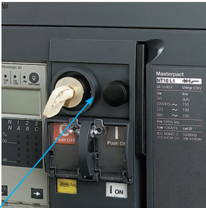
Electrical closing pushbutton BPFE.
